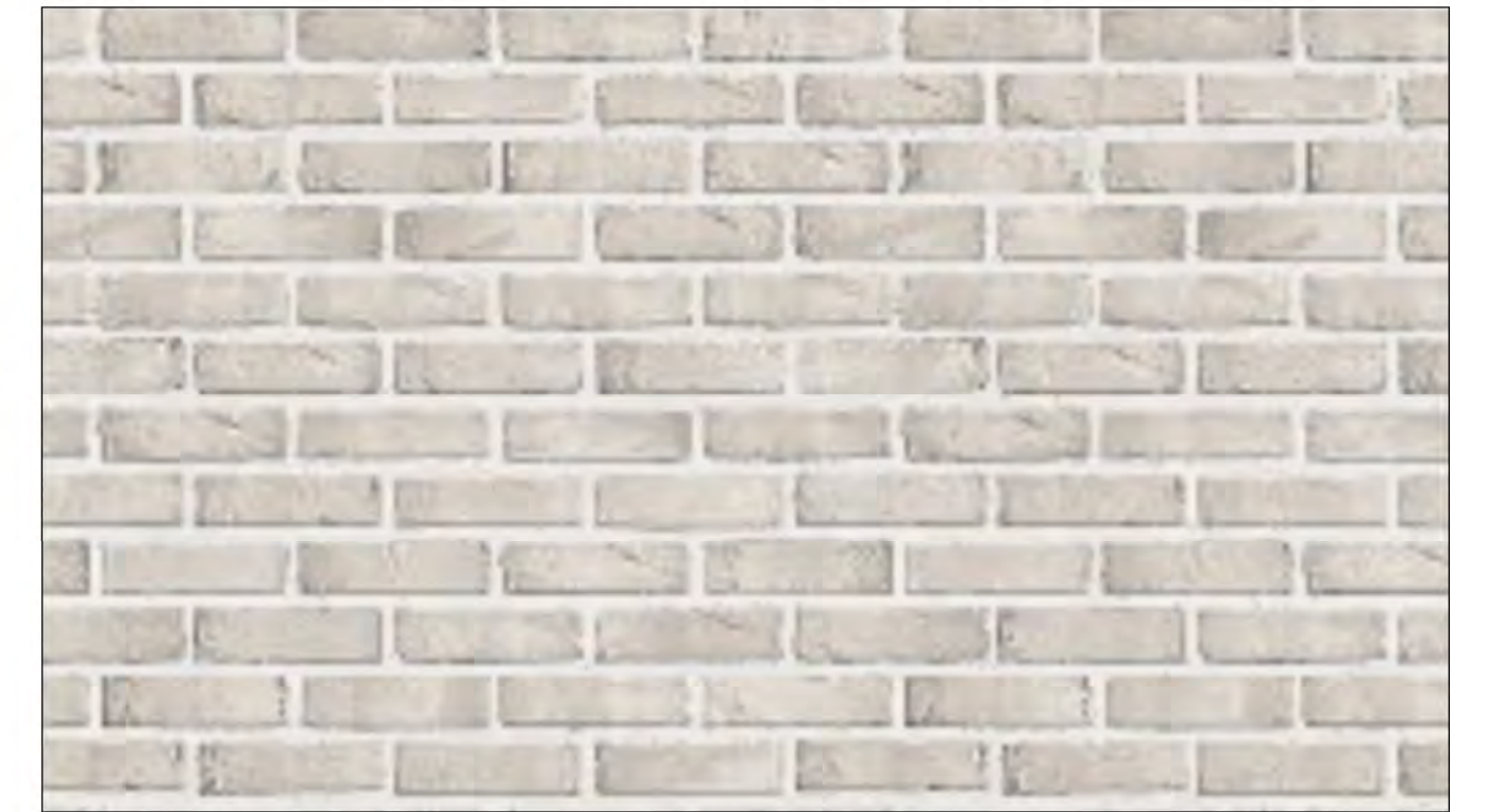
Stretcher bond brickwork
