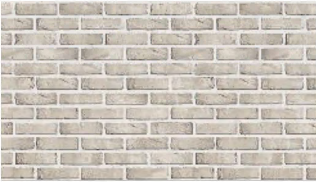
Stretcher bond brickwork
