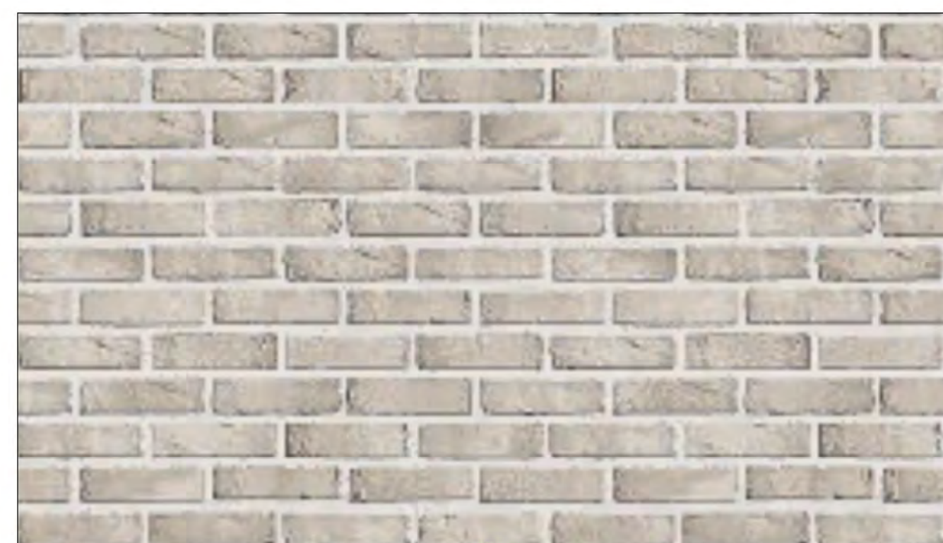
Stretcher bond brickwork
