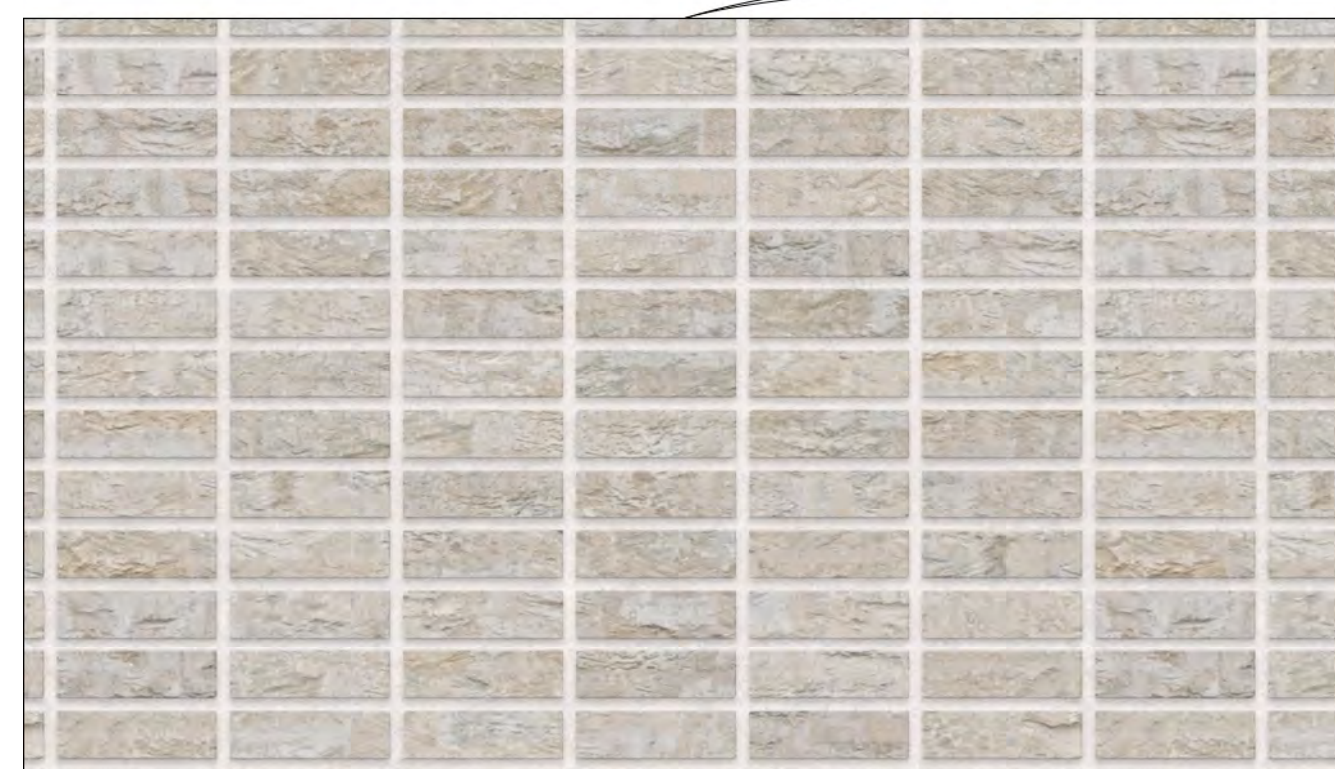
Stack bond brickwork
