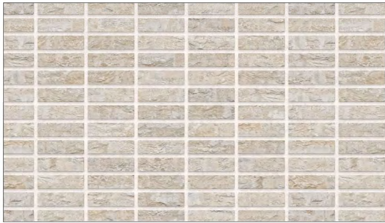
Stack bond brickwork
