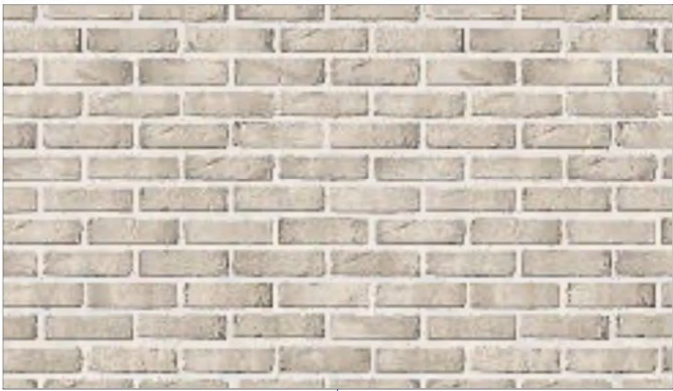
Stretcher bond brickwork
