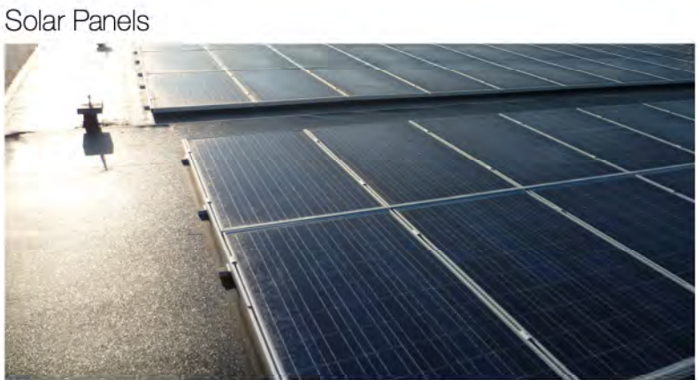
Solar Panels laid flat on stub legs/rail system
