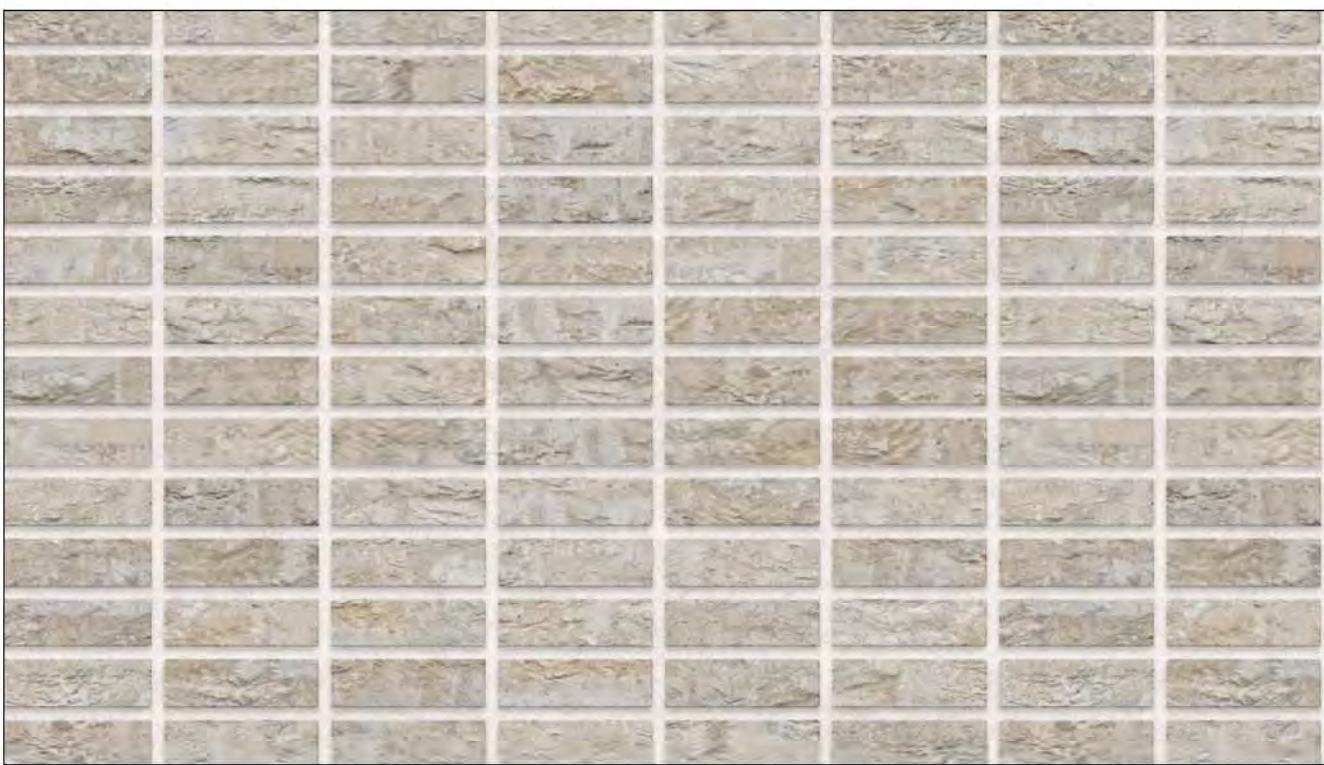
Stack bond brickwork
